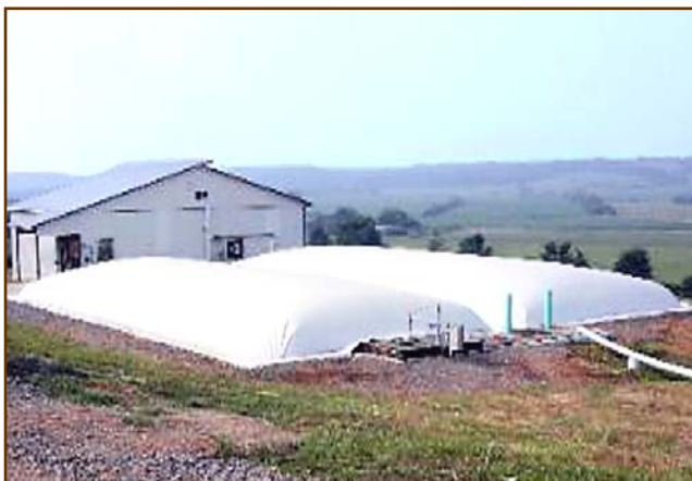
Figure 1 A medium-scale on-farm “covered lagoon” biogas facility for manure on a US dairy farm.
